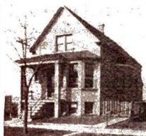
A No. 2118 IDEAL Boiler and 270 ft. of 38-in. AMERICAN Radiators, costing owner $135, were used to Hot-Water heat this cottage.
